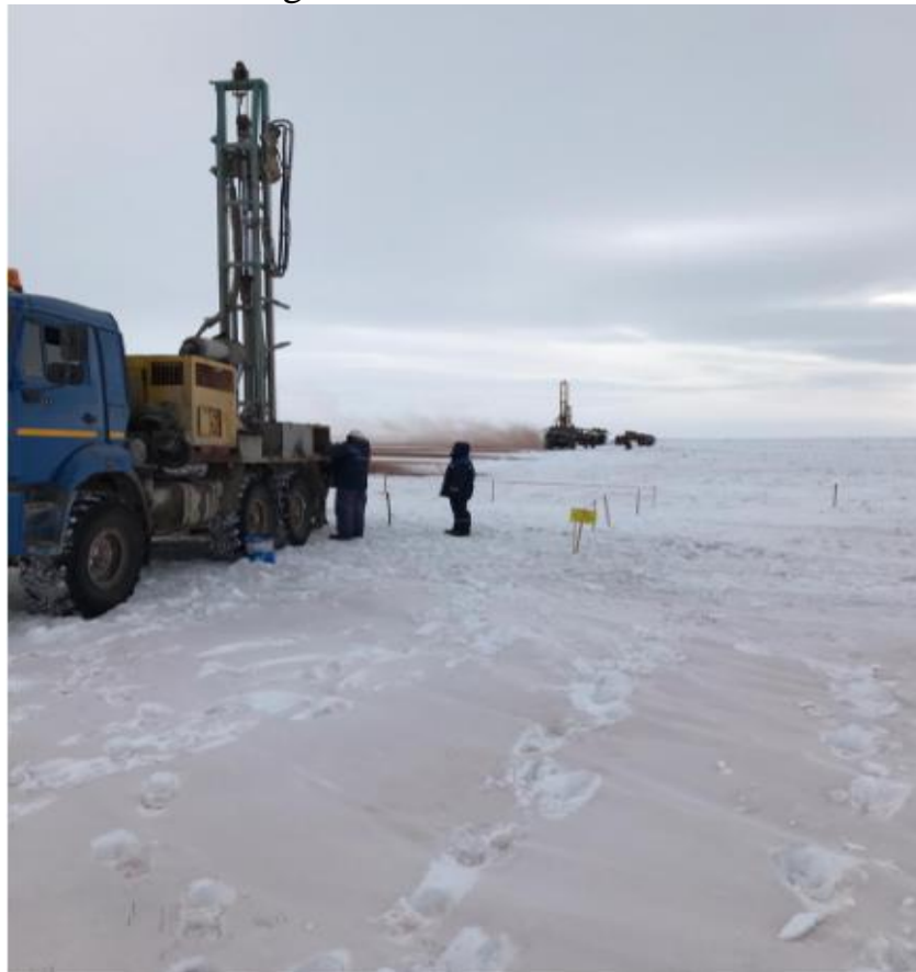
Figure 3.3.3.1 – Drilling of a well under an explosion at a SP
